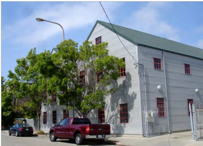
The Light Industrial zone is up to two stories in height, and is occupied by industrial, manufacturing, office and small scale retail uses.
