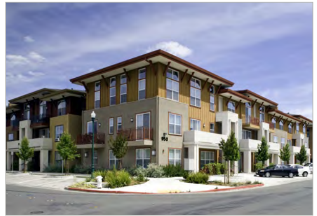
Example of a building that breaks up the Primary and Side Street façades into different vertical components by projecting or recessing external wall surfaces and by adding porches, balconies, etc..
