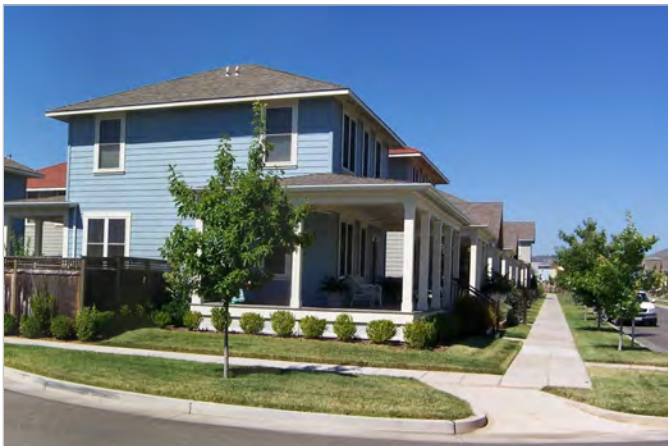
Example of a building that incorporates the same materials and finishes on both its Primary Street and Side Street façades. Its front porch also faces both streets.
